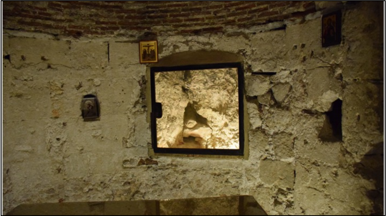
Traditional crack that formed with the earthquake upon the death of Jesus (Matt 27:51). This is downstairs under "Golgotha."
